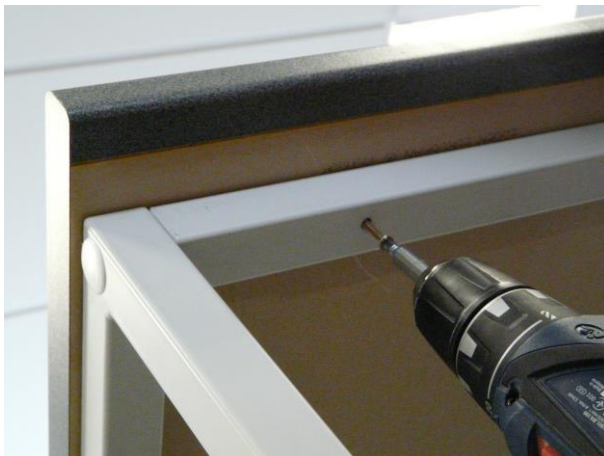
17. Screw the frame with worktop
